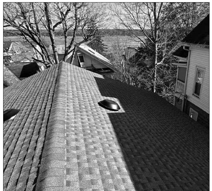
The new Westervelt roof will protect the building for decades.
