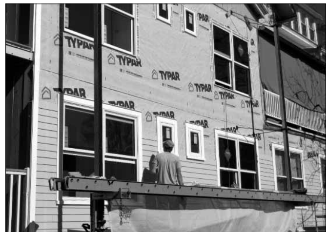
A workman installs new siding and windows on the Shaw building.
